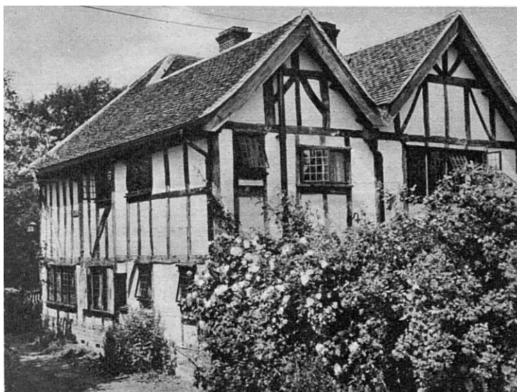
The side and rear elevations prior to alterations. alterations (Illustrated Sporting and Dramatic News, 1st October 1951)
