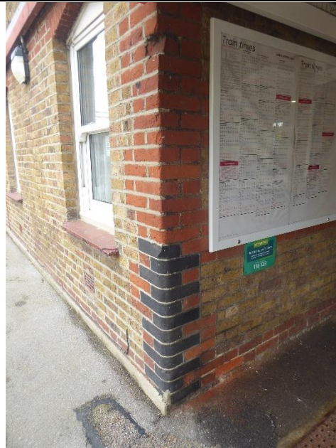
Detail of black bullnosed bricks to platform
