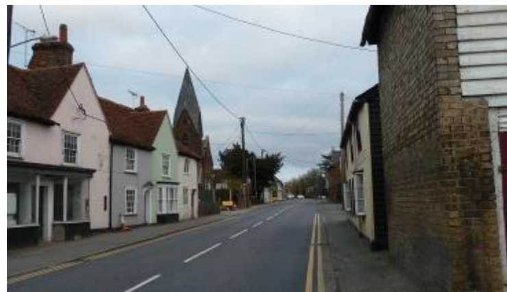
The Street, Hatfield Peverel 2016
