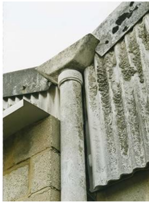
Asbestos cement downpipe, hopper and profile sheet
