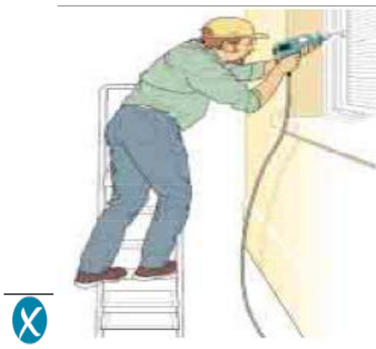
Incorrect – steps side on to work activity
