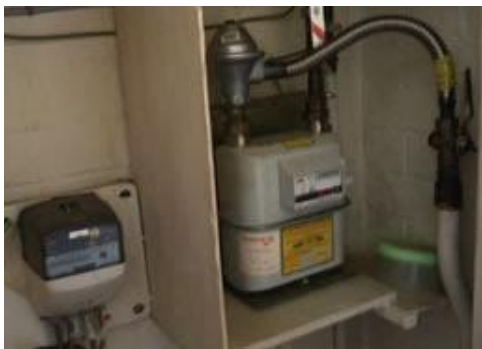
Asbestos panelling around a gas meter
