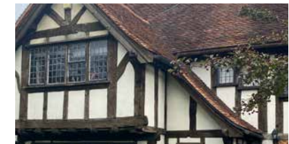
Half timber framing (mock tudor facade) with white render.
