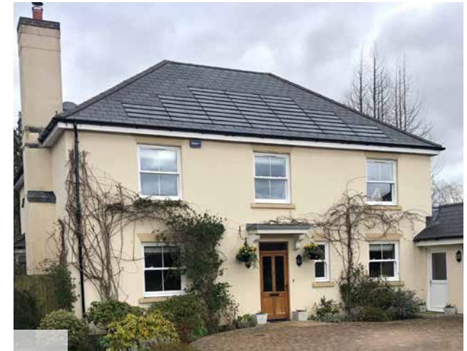
Figure 84: Use of shingle-like solar panels on a slate roof, with the design and colour of the solar panels matching those of the adjacent slate tiles.
