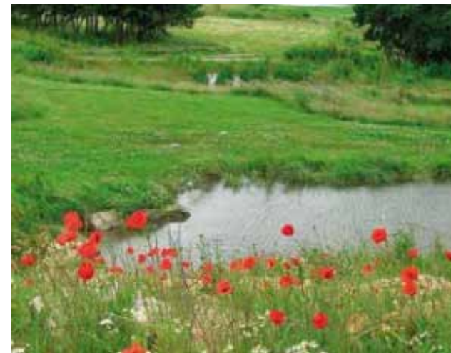
Figure 13: Manor Park, Sheffield – the first of three basins in the foreground collecting runoff from 300 houses
