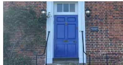
Georgian doorway, with flat top pediment and wood pilasters and typical 6 panel solid wood painted door, with vertical fanlight.
