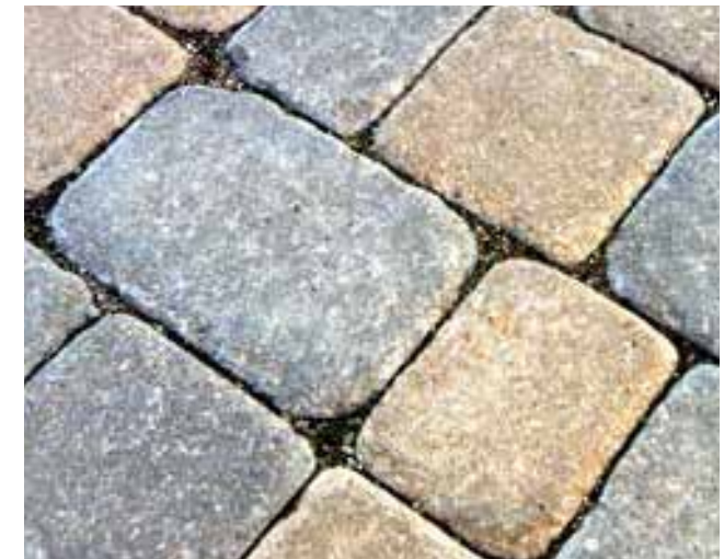
Figure 68: Example of a permeable paving.
