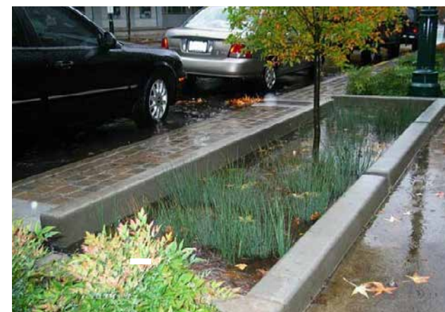
Figure 14: Example of sustainable drainage incorporated into the street scene.
