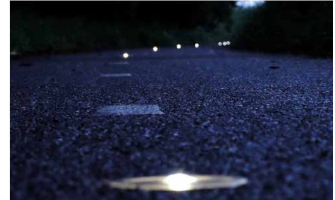
Figure 47: Example of a foot/cycle path which is lit by solar cat's-eye providing some light for pedestrian and cyclists without creating any disturbance to the nearby properties or unacceptable levels of light pollution.
