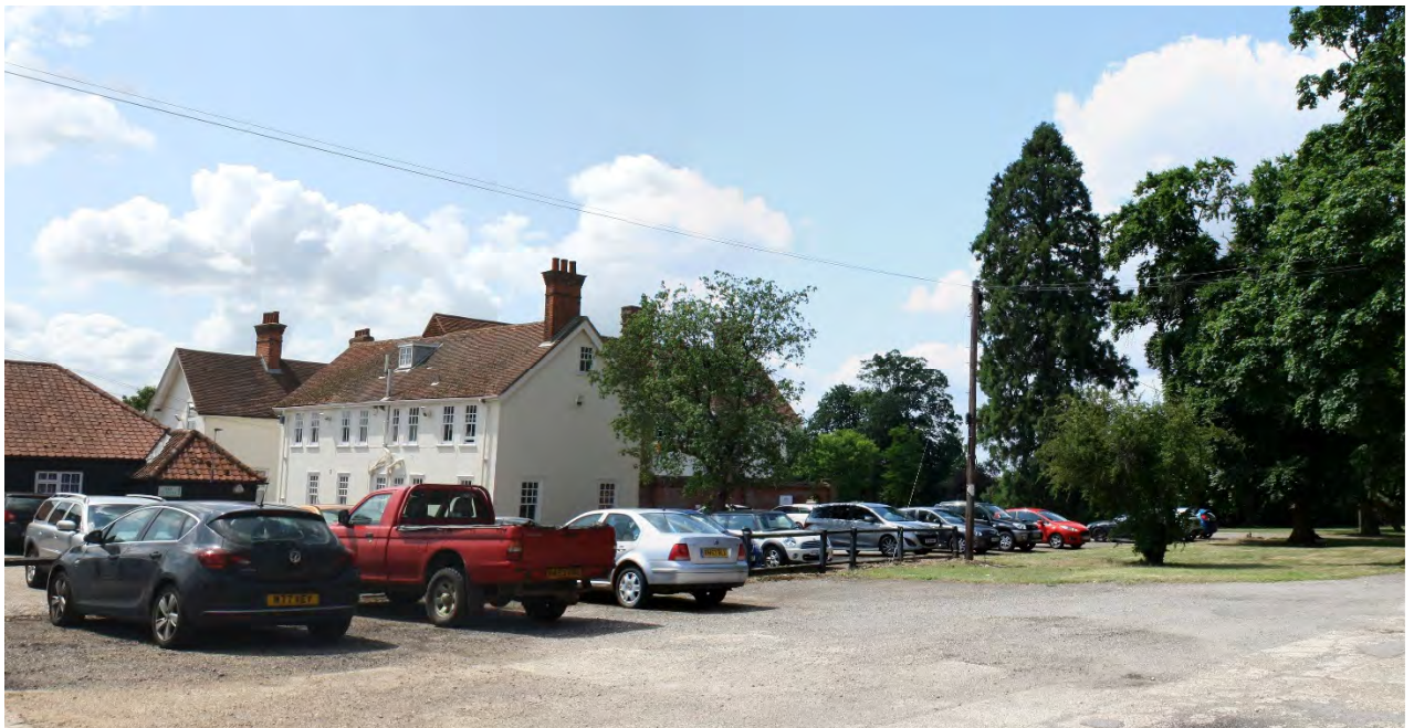
Farmstead and businesses at Whitelands on the Terling Road
