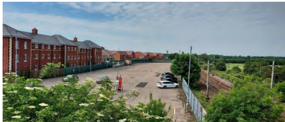
Station Car Park
